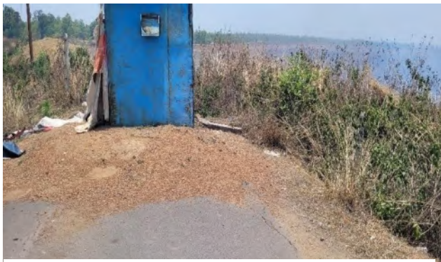
Current Condition the Intervention at Intervention Site
