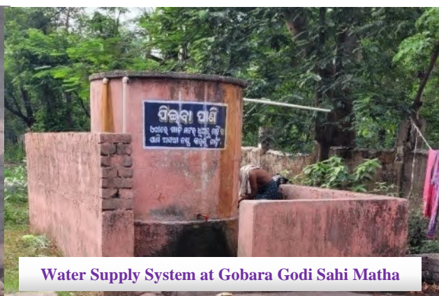
Pipe Water Supply System at Gobara Godi Sahi Matha
