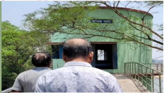
Intake Well at Santhapada
