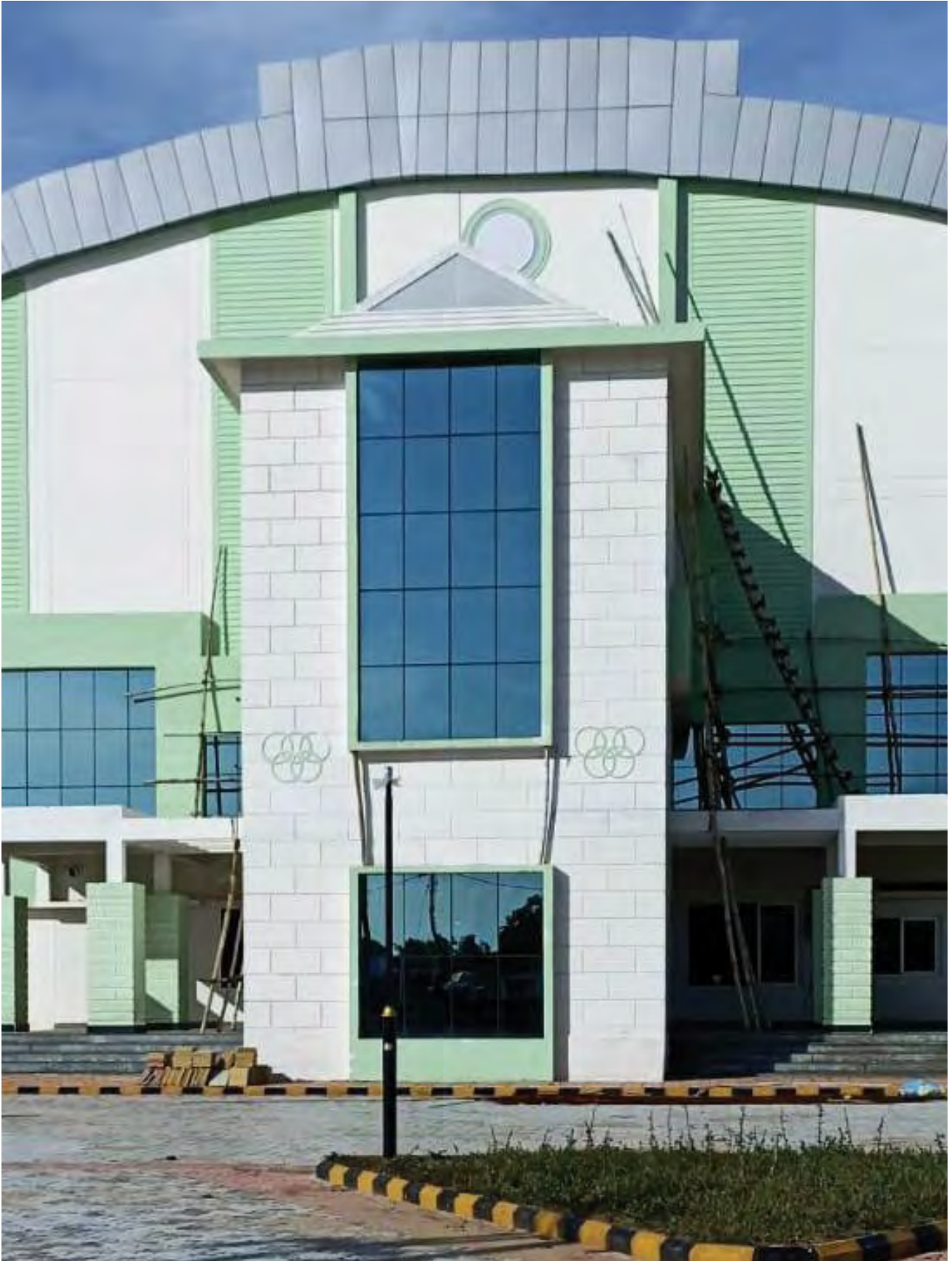
Multipurpose indoor stadium, Jajpur
